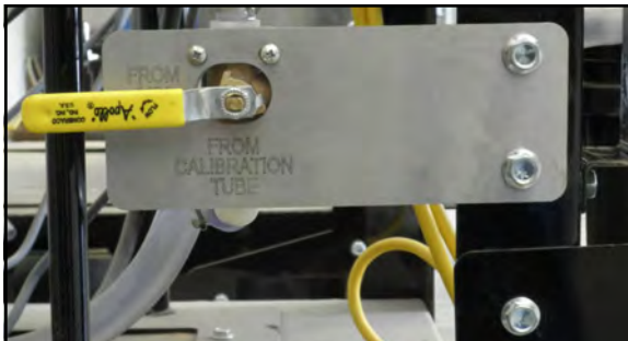
Drawing chemical from the bottom of the Mix Tank
