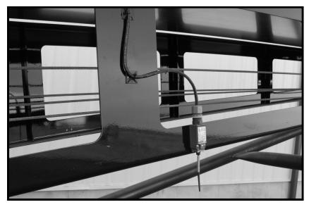
Picture of the limit switch after installation.
