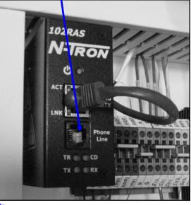
14. Connect a dedicated analog phone line to the modem located in the top left portion of the control panel. This will allow USC remote access to the seed treater to help diagnose and fix problems that may arise.
